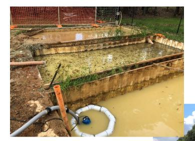
Liquid waste from drilling operation
